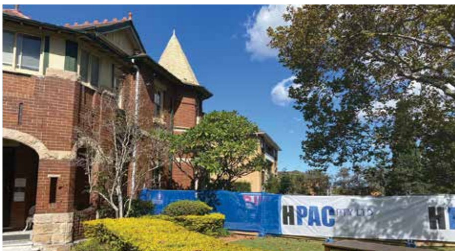
Early works commenced at Tresillian Wollstonecraft in March, 2021.
